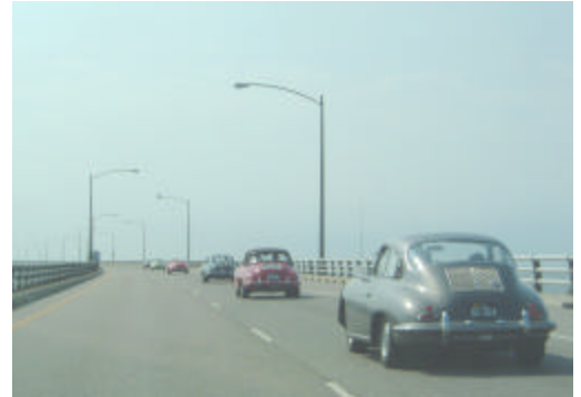
Chesapeake Bridge Tunnel (Photo by Swenson)
